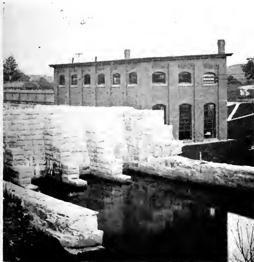
FIG. 6.—BIRCHEM BEND CANAL AND TAIL-RACE, SPRINGFIELD, MASS., PLANT.
